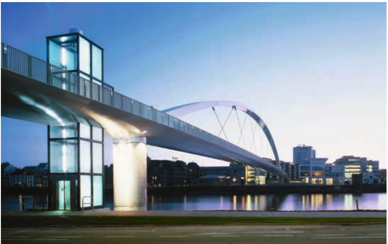
The new pedestrian/cycle bridge links the Céramique district with the centre of Maastricht. The bridge was largely financed by Vesteda/ABP as part of the Céramique public-private partnership.
