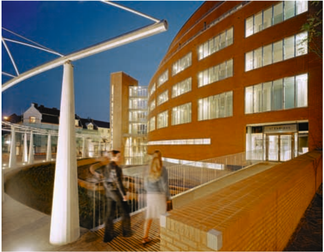
Public space for the Céramique Health Club, Cortile project, Maastricht
