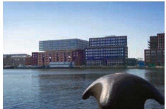
Detroit contains 81 comfortable loft apartments, ranging from 106 m 2 to 238 m 2 . The apartments can be arranged at will; a single large space, or perhaps a more traditional arrangement of, say, three bedrooms. The penthouses in Detroit have roof terraces of 120 m 2 offering views over the IJ.
